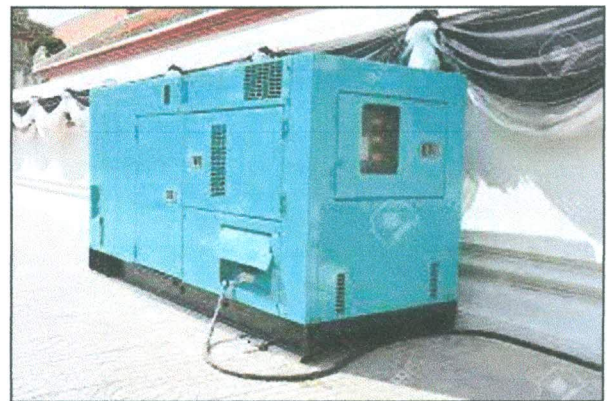
Fig-1: Emergency Diesel Generator (EDG) with canopy made up of sheet metal
